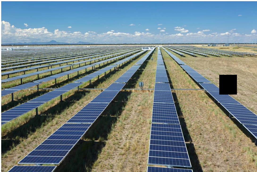
Plate 3-2: Single-axis Tracker Arrays
